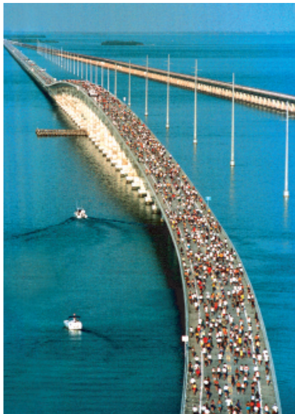
A marathon being held on Seven-Mile Bridge in Marathon, Fla.
