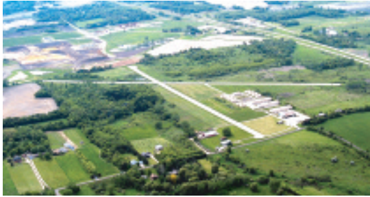
A new industrial park is located west of Blackhawk Airfield, Cottage Grove, Wisconsin.
